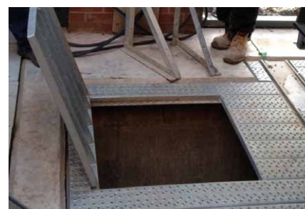
Practical access to the pit
